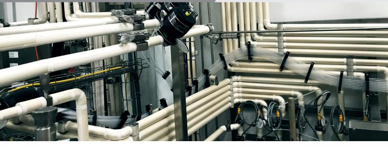
It seems obvious that increasing the thickness of an insulation material will reduce the heat loss from the pipe that it is insulating. But what happens if pipework is too densely packed, and using a thick insulation actually prevents certain parts of the pipe being insulated?
