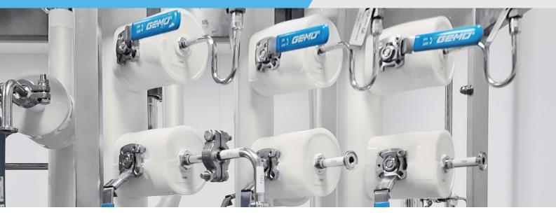
T-FIT® Clean insulation is developed from Zotefoams' ZOTEK® F 42 HT LS PVDF closed cell foam, a material which has numerous benefits when it comes to insulation, especially within Pharma, Biotech and Semiconductor cleanroom environments.
