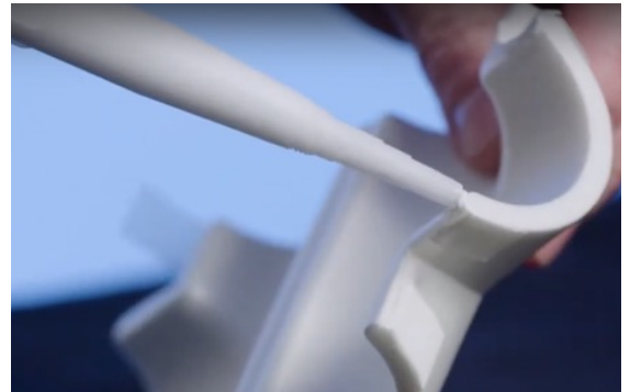
5.2 Carefully apply sealant to the fitting edges.
