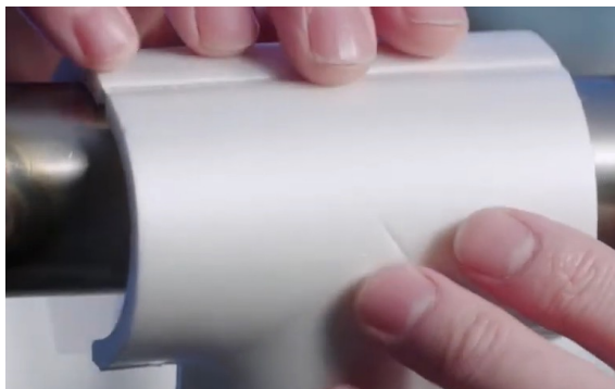
5.3 Install the prepared tee fitting.
